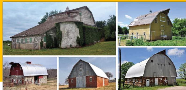
The historic survey of barns identified some beautiful structures like the ones shown here in every region of the state.
