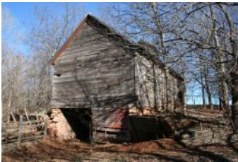
Left: Small (24' x 40'), three-level timber-supported, gable-end bank barn with cupola, in the Cordell vicinity, central Washita County (ca. 1900). Trap doors in the granary open to mangers in the south-facing basement stock pen. This notable building lies squarely within a Railroad-recruited Volga German colony. Its form follows no known Pennsylvanian precedent and may represent a direct Old World transplant.
