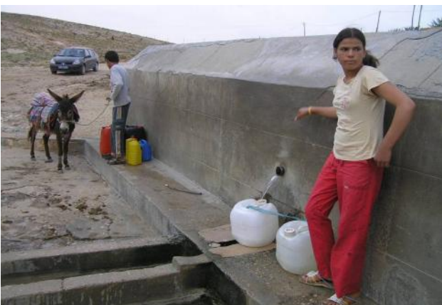
Left: Public water tap constructed at the exit of a still-active qanat.
